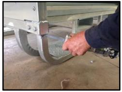
**STEP 80:** Fully tighten bolts and nuts connecting posts to base. Selastic the bottom of the posts to the frame so they are water proof.
