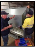
**STEP 64:** Always tek screw top of the flat side first. \*\*Put side with 4 holes on top, on the same side as lid hinges.
