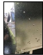
**STEP 5:** Don't tek screw this side of ends. This will be done when rain guards are fitted later.
