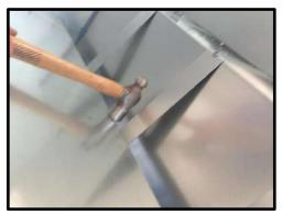
**STEP 37:** If divider needs straightening so straps line up, always hammer on corners.
