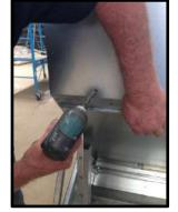
**STEP 65:** Second tek screw to be the second hole from the end (Do not do the hole at the end first).
