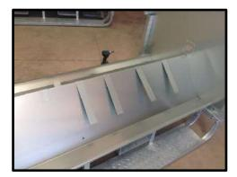
STEP 23: Lay out straps on top of base.
