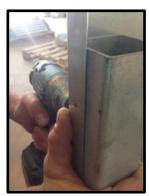
**STEP 6:** Ensure post and edge of end are fitted with no gap. Tek screw ends fully to posts.
