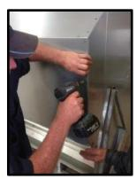
**STEP 66:** Tek screw the bottom bend then tek screw the side completely to feeder (Do not miss any holes).
