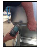
**STEP 68:** Tek screw second hole from the end. Do not do first hole first.
