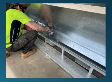
Tighten the 7 tek screws on top of the base sheet to connecting the straps to the base
