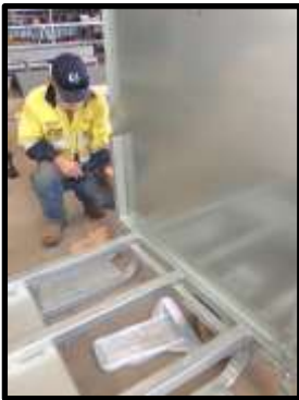
STEP 4: Connect ends to frame.
