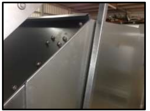
STEP 78: If only attaching one pad bolt place tek screws in holes not used on the other side.
