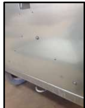
STEP 12: Tek screw to ends.
