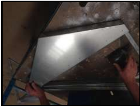
STEP 40: Pull down firmly and screw.
