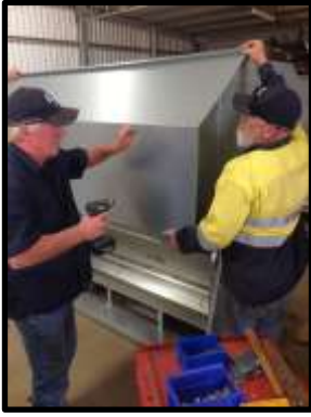
STEP 61: Always tek screw top of the flat side first.
