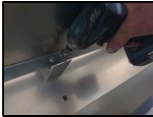
STEP 32: Two screws per strap.
