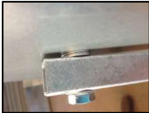
STEP 43: Attach lid hinge to end, one washer between bolt and RHS, three washers between RHS and end.
