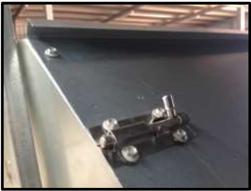
STEP 76: Attach pad bolt to top of the side (Use second holes from top, the bottom hole to be drilled).
