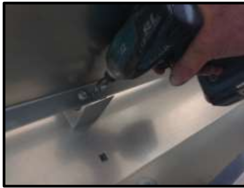
STEP 32: Two screws per strap.
