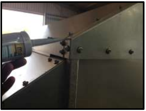
STEP 79: Sealastic all areas that are exposed to water.
