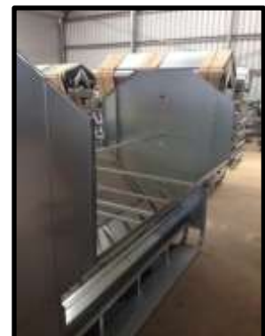
STEP 60: Feeder is now ready for sides.
