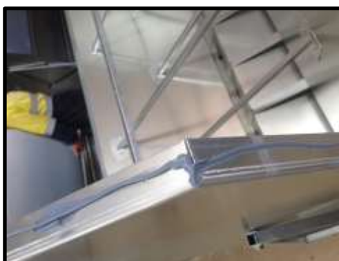
STEP 59: Be sure to silicon all gaps.
