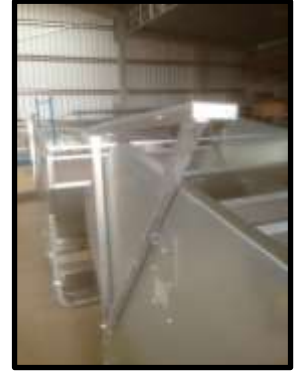
STEP 81: Attach bridging piece to RHS hinge.
