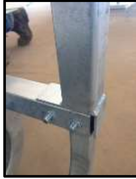
STEP 2: Connect post to frame. Ensure flat washer is put in front of nut.
