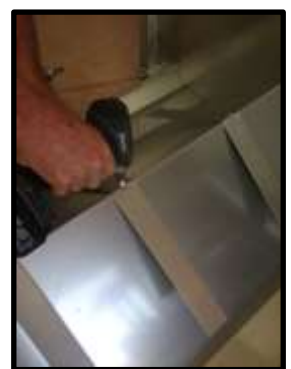
STEP 21: Fit the seven straps to base. Holes located at the top of the bend of the base.
