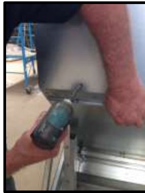
STEP 65: Tek screw second hole from the end. Do not do first hole first.
