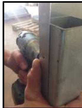
STEP 5: Ensure post and edge of end are fitted with no gap. Tek screw ends fully to posts.
