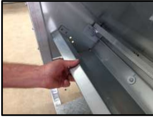
STEP 50: Attach bottom adjuster (Has 3 slots).
