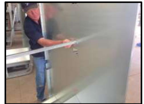
STEP 9: Connecting main support.
