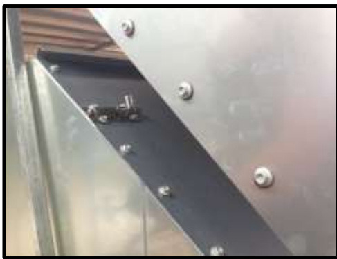
STEP 77: Pad bolt attached.
